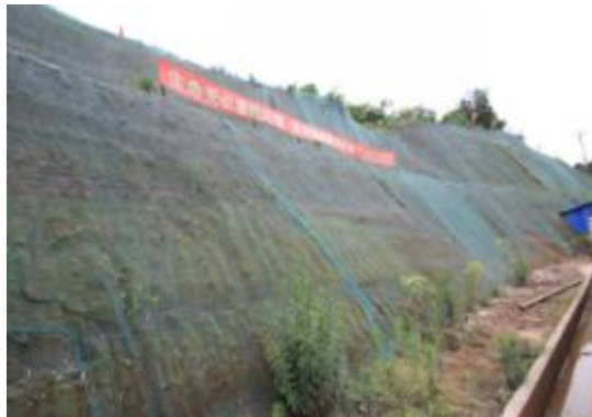
ZCB4 拌和站边坡遮盖
