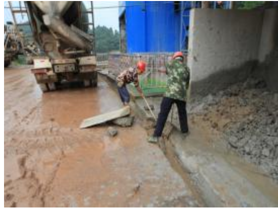
ZCB3 拌和站清理压滤渣
